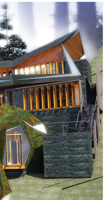
The overall form is envisaged to simulate a cavernous space or an ant hill, sporadically deriving its form from nature. The cottage pods and the roof for the main building have been designed as a composite structure using a skeleton of tubular steel framework covered with thin ferrocement shell. The austere skin of the roof gets a natural makeover by the local flora taking over and imitating like giant moss covered rocks in a forest.
