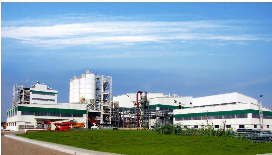
Wet Mill and Refinery buildings are connected by Services Building. Both these buildings are having two mezzanine floors each, with each floor in both the buildings loaded with heavy equipments ranging from 20 MT to 100 MT with dynamic operations, and collateral load of 100 kg per square meter
